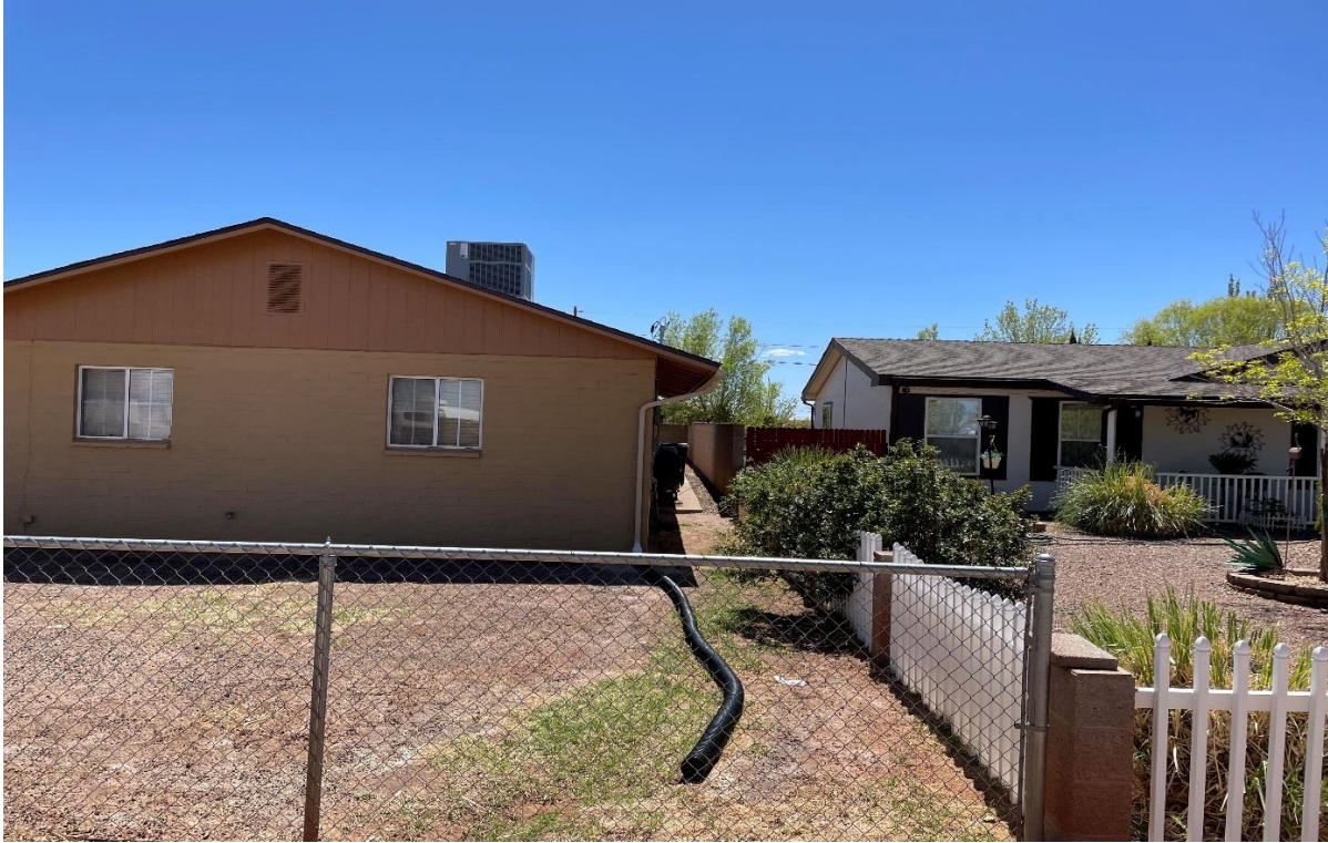
Picture shows lack of the rear yard at 521 North Pope Avenue.
